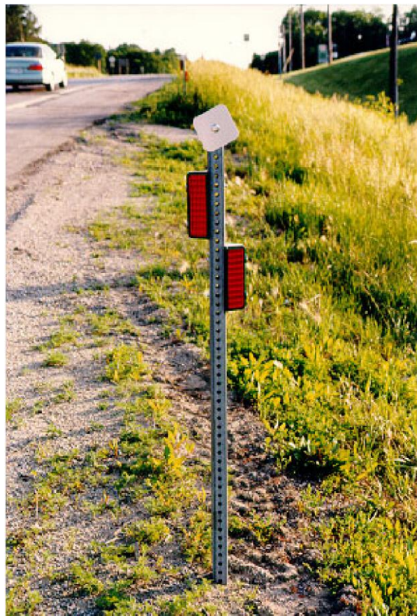
Alternate Back-to-Back mounting method using Telespar posts
