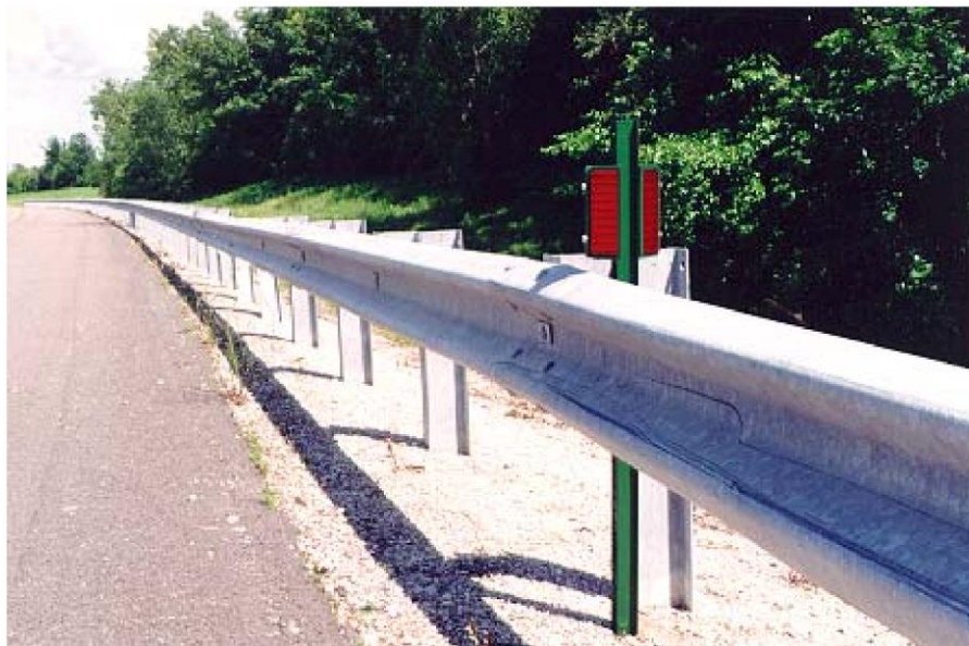
Example of Reflector Installation where guard rails are present
