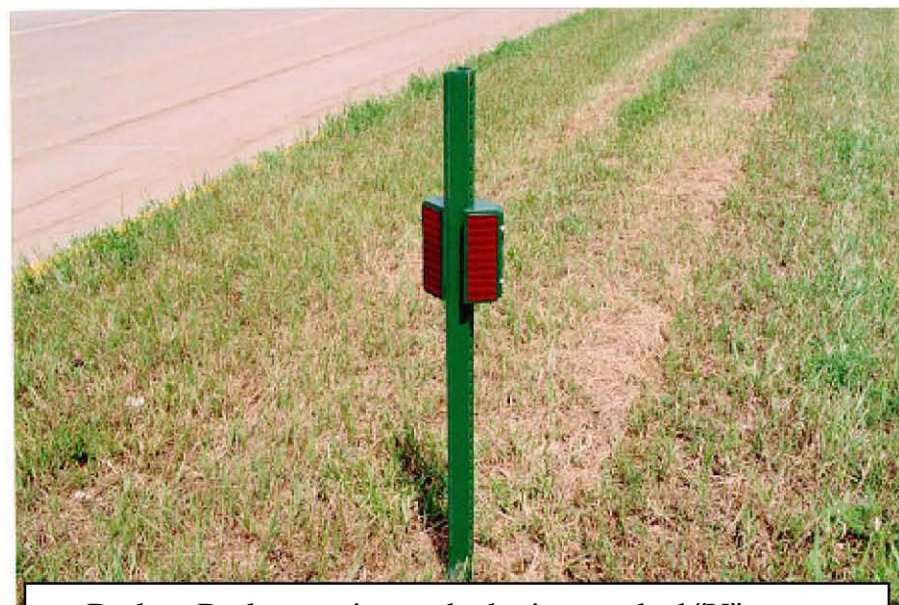
Back-to-Back mounting method using standard "U" posts
