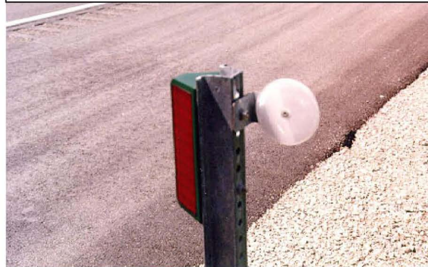
Single mounting method using standard "U" posts
